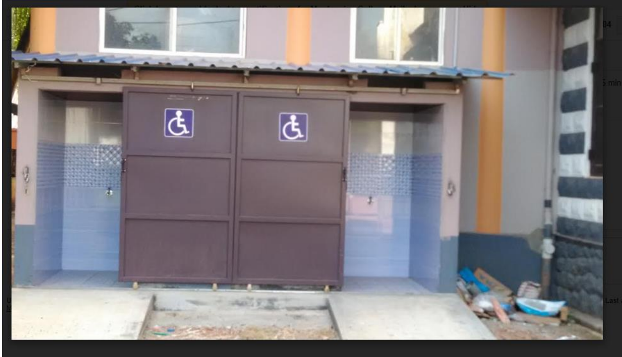
Separate toilet to boys and girls and Ramp access towards the toilets
