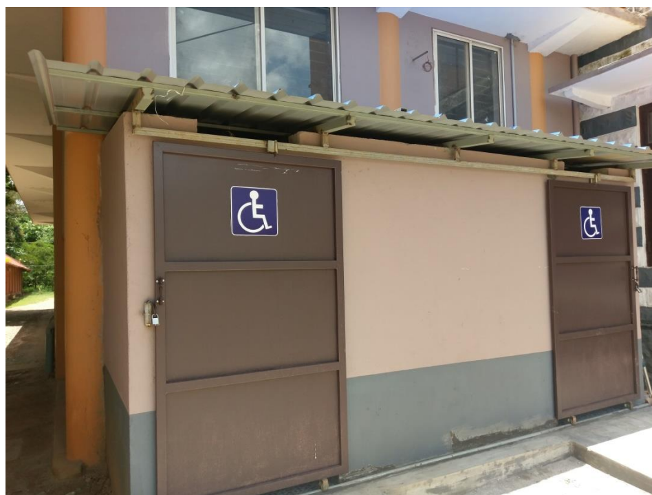
Accessible toilet and changing facilities located in the campus; a wheelchair accessible toilet provided for girls' and boys' toilet separately
